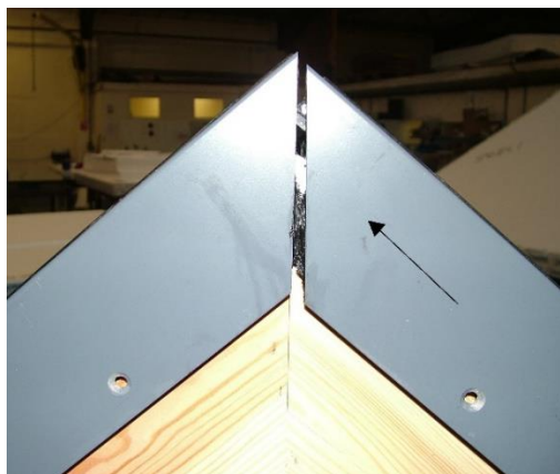
Figure 11 – The second section is pushed up to meet the first section at the apex
