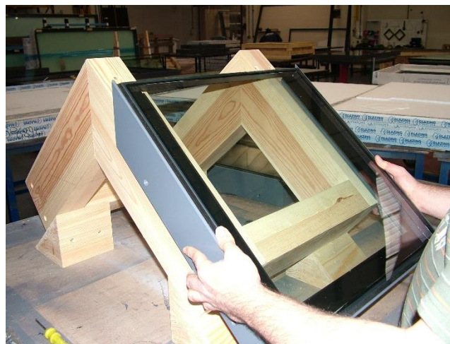
Figure 8 – Installing the first half of the unit
