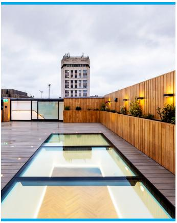
On this particular project, the sliding section when open provides a clear opening of 1927mm on the left side when viewed from the outside and is glazed on the front and top with a built-in fall of 3 degrees, and mounted to walls at the rear and two sides. The skylight also includes the optional extras of a proximity detector and a battery back up. The skylight was crane lifted to the roof so that installation could be carried out.
